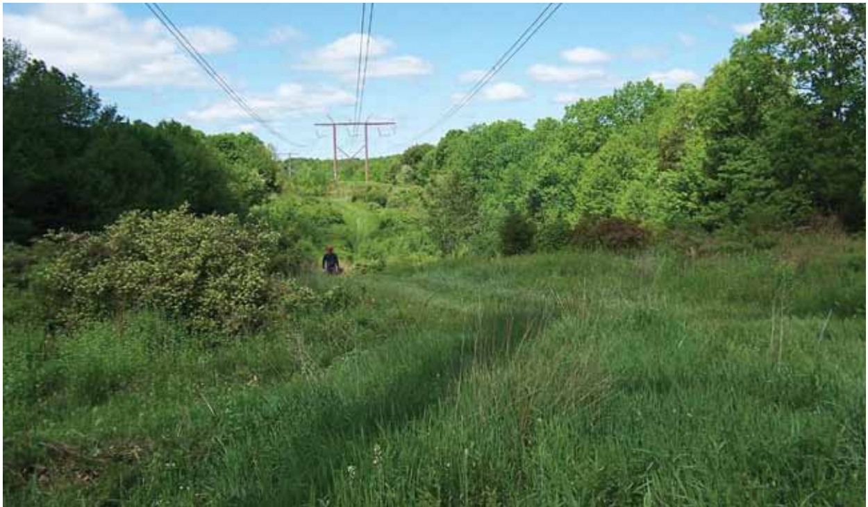
NYPA manages the Marcy South transmission right-of-way using principles of integrated vegetation management.
